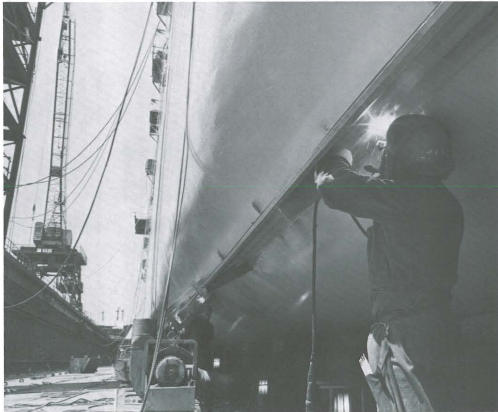
Welders complete the addition of bilge keels, which run the length of each side of the ship at the turn of the bilges. The keels will provide added stability by reducing ship roll underway.
